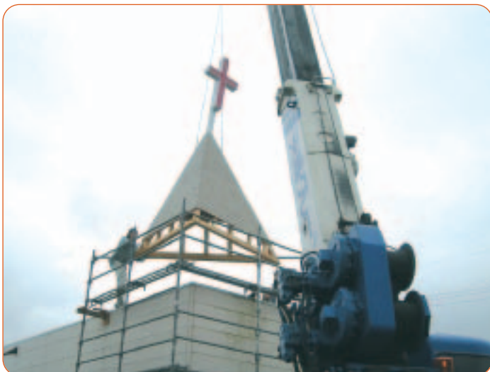
Crowning the new church in Takamatsu
